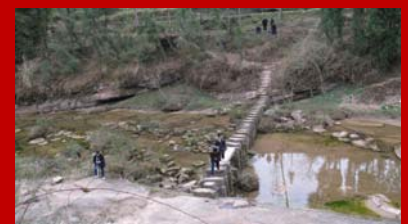
Original stone bridge in Baofeng Village
