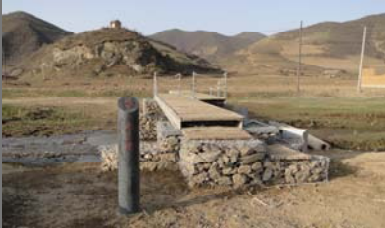
The second WZQ in Datan Village was successfully built
