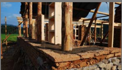
The construction of the key wall structure is in progress
