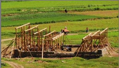
An external timber framework was built by villagers within a day
